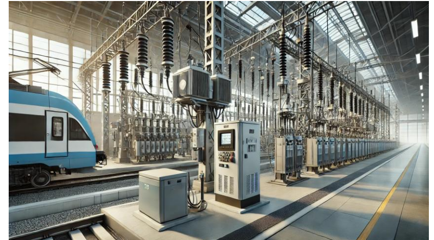
Electrical Stationary Equipment and Infrastructure
